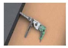
Then drill and fix deformed bars (ø16 x 600 lg) in each concrete slab. At least 3 dowels per meter in each concrete slab. 300 mm of the dowel must be fixed in the concrete (ideally with resin anchorage system) and 300 mm must stick out. Put also special primer on all vertical sides of the concrete slab.
