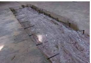
Install a HC Sinus Slide® joint in the middle of the gap opening between the concrete slabs. Level out the HC Sinus Side® joints down and across. Eventually, weld the dowels fixed in the concrete slabs to the anchorage system of the HC Sinus Slide joint or use reinforcing mesh to link dowels and joint connectors.
